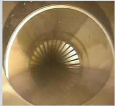
Broken joint in relief well collector system pipe
