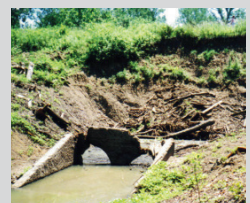
Outlet and embankment collapse
